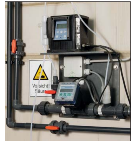
Correct acid dosing thanks to pH-value measurements
